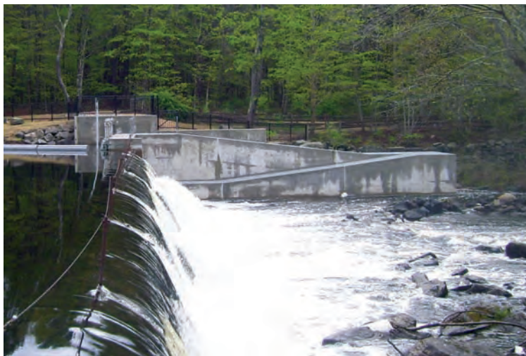
Newly installed Wiswall Fish Ladder on the Lamprey River, Durham, NH. Photo by D. Cedarholm
