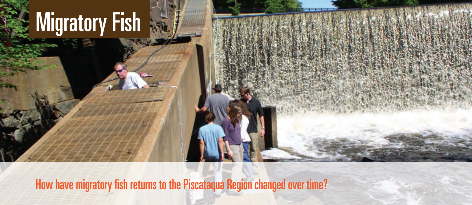
Fish ladder on the Lamprey River, Newmarket, NH. Photo by PREP
